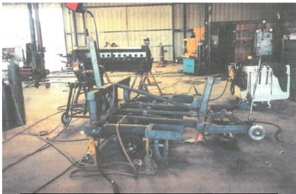
Main frame Construction
